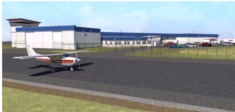
Ground-level View of Commercial High Altitude Balloon Flight Facility (Above)
